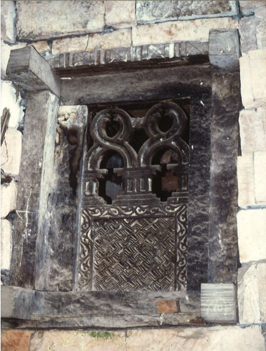
One of the three windows at the backside of the Church
