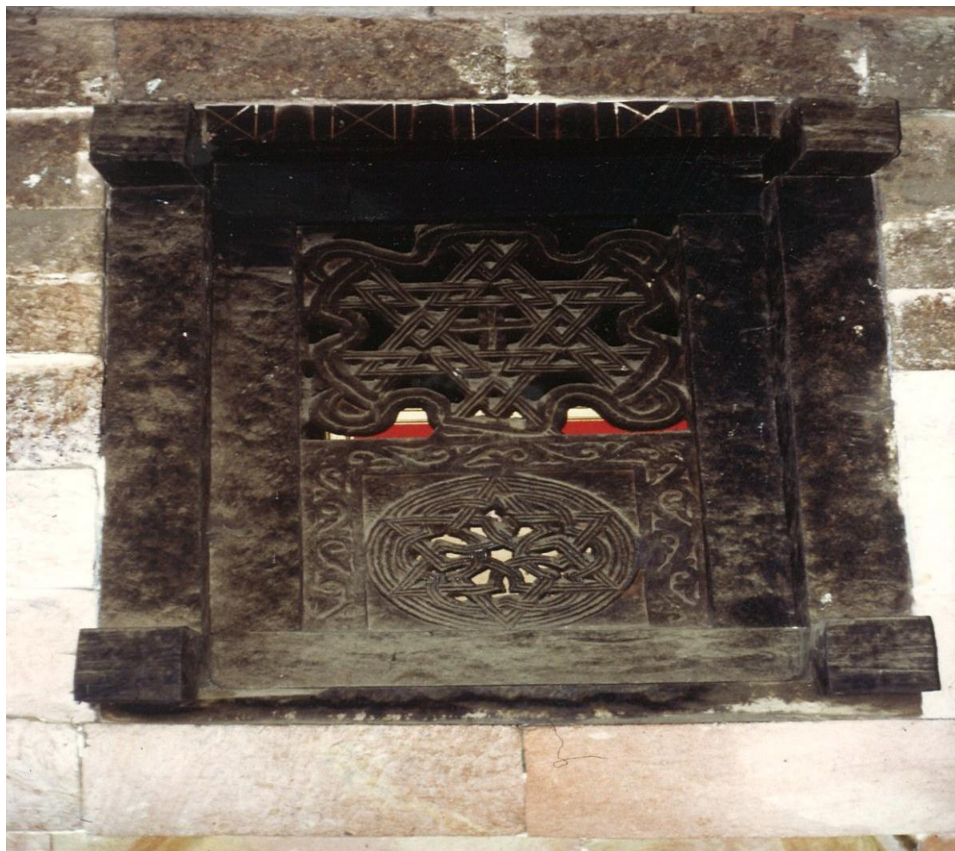
One of the three windows at the backside of the Church
